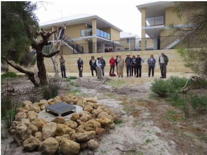
Stormwater from the housing units in the background is directed into the bushland via a bubble-up pit in the foreground. Photograph courtesy of M Radestock CRREPA
