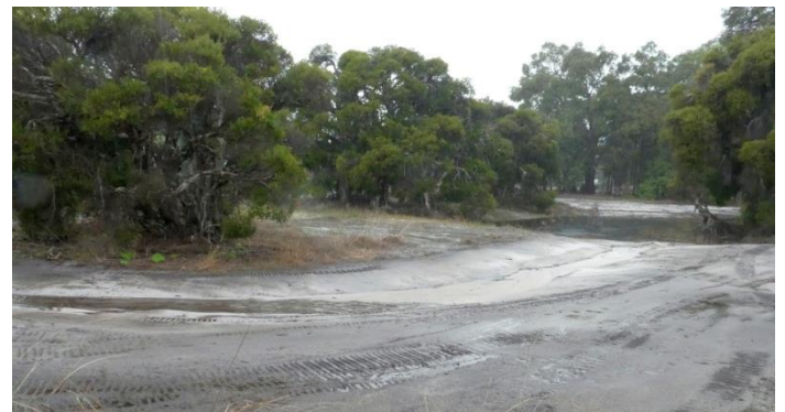
Stormwater flows from the road (left, out of shot) into the depression.
