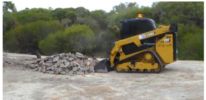
The rubble was picked up by a skid steer and placed in a truck.
