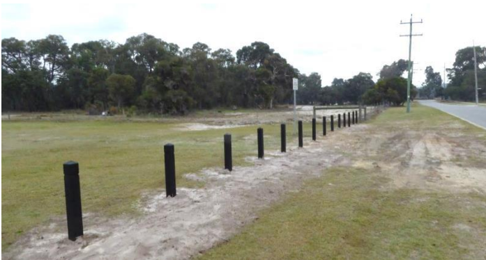
Bollards along Gibbs St adding to the protection of the bushland.
