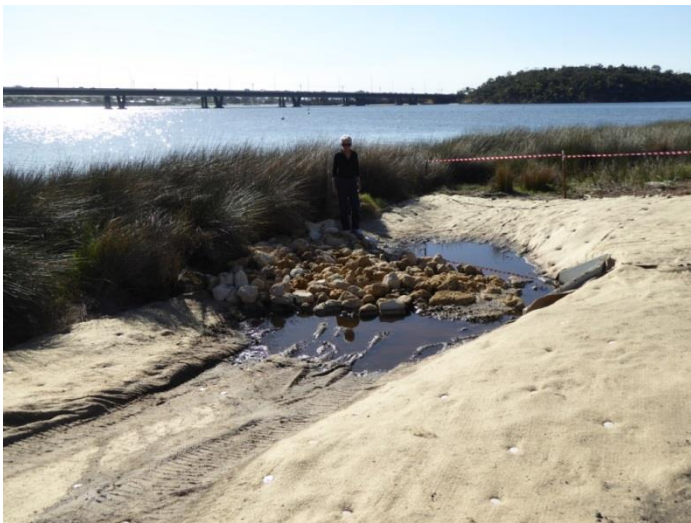
Newly constructed living drain. Photo courtesy of CRREPA - Colma
