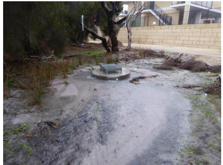
Water flows from the houses behind to the bubble-up pit in the bushland.
