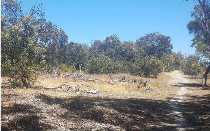
Before the bricks were removed. The piles of bricks had been there so long that they had been covered by leaf litter, weeds and dead branches. Photo: Shaun from A Bobcat Service.
