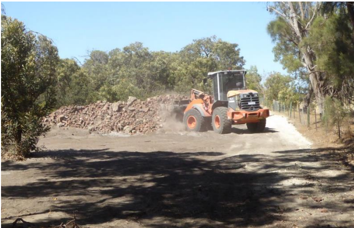
A loader was used to get the bricks onto the trucks.
