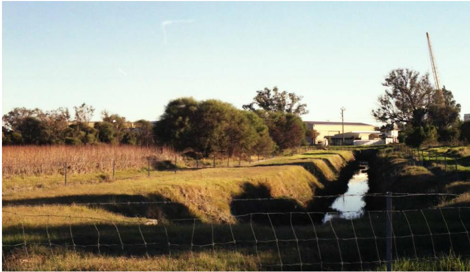
Left - Standing on Station Street, looking along the straight drain towards Welshpool Road.
