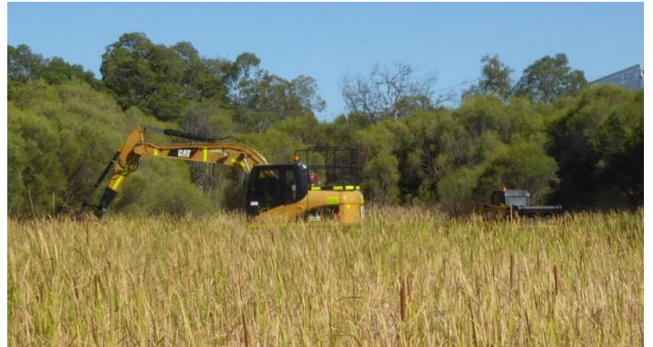
An excavator scrapes the basin clean.
