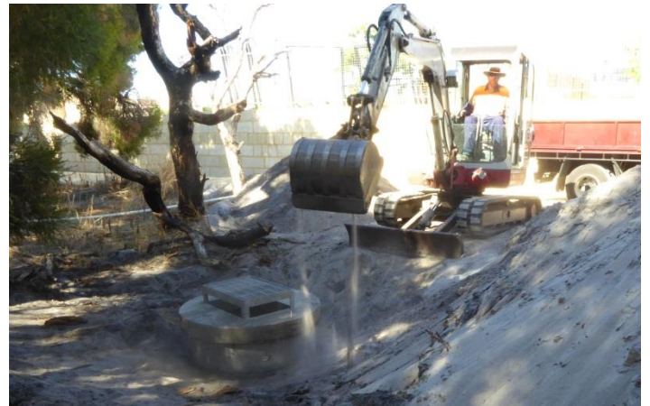
The bubble-up pit is installed.
