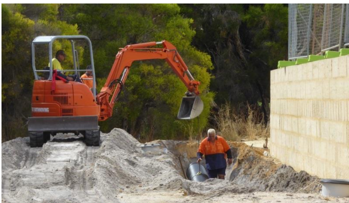
Stormwater pipes are laid from the housing development to the bushland.
